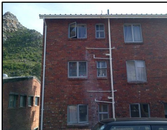
Fig 2. Renovated flats at Waterfall Barracks.
